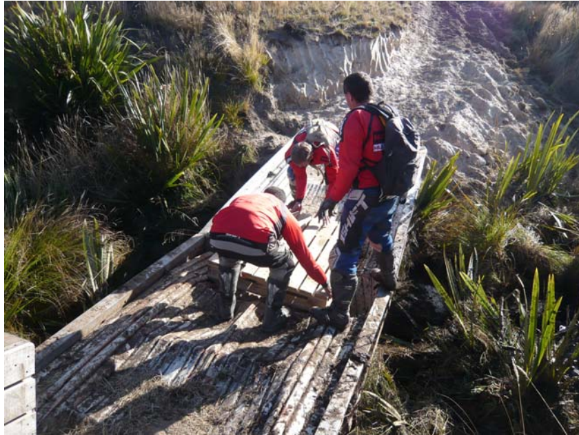
Emergency repairs to bridge 1
